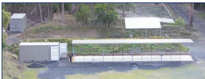
New facilities at the MR have led to impressive growth in use.
